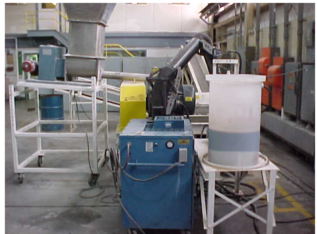
Photo 2 – Feeding and Binder Tank
